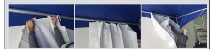
Starting from the middle of the frame feed the right hand side of the wall towards the right leg. Keep feeding all the tabs and drag the wall across.
