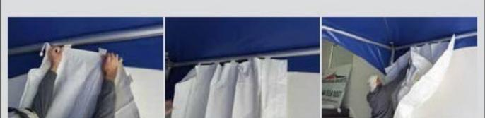
Starting from the middle of the frame feed the left hand side of the wall towards the left leg. Keep feeding all the tabs and drag the wall across.
